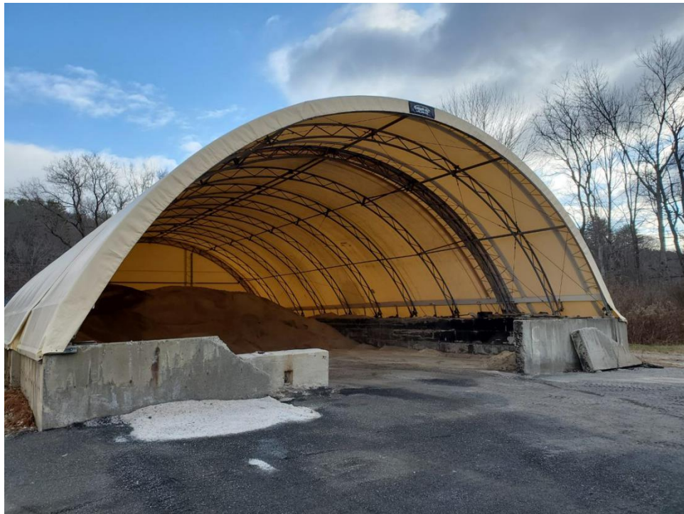
Figure 1: Front of Existing Salt Shed
